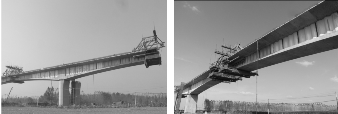
Figure7, Photos of cantilever construction.
